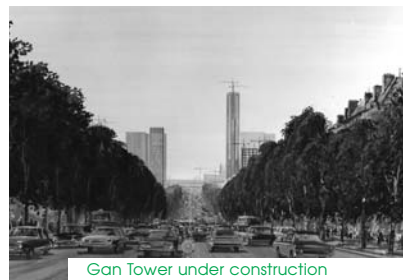
Can Tower under construction
