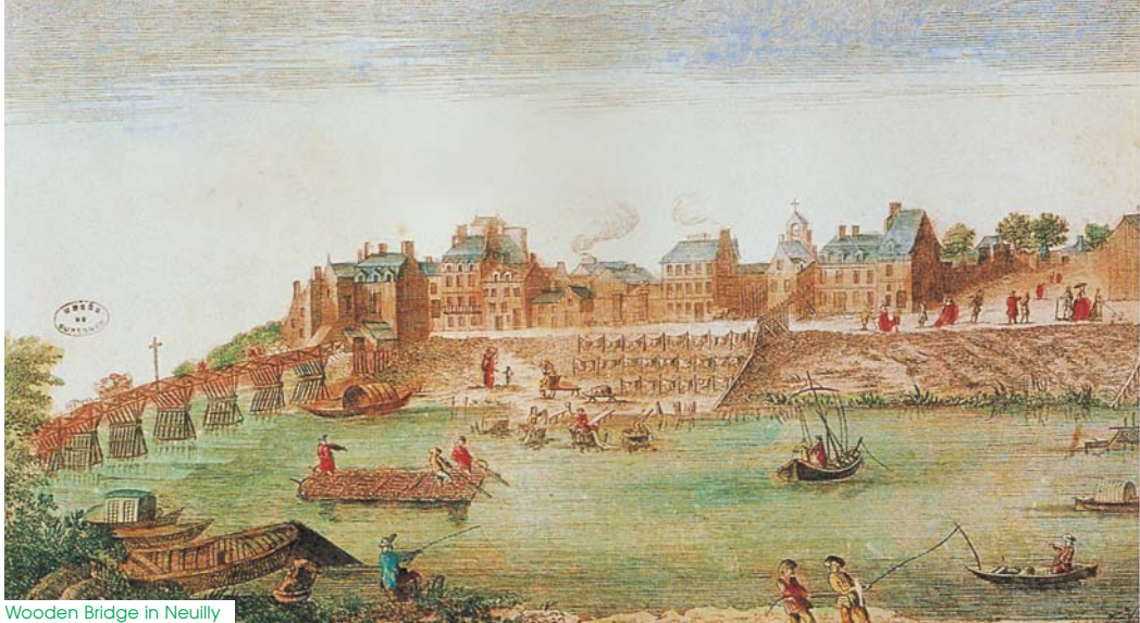
Wooden Bridge in Neuilly
