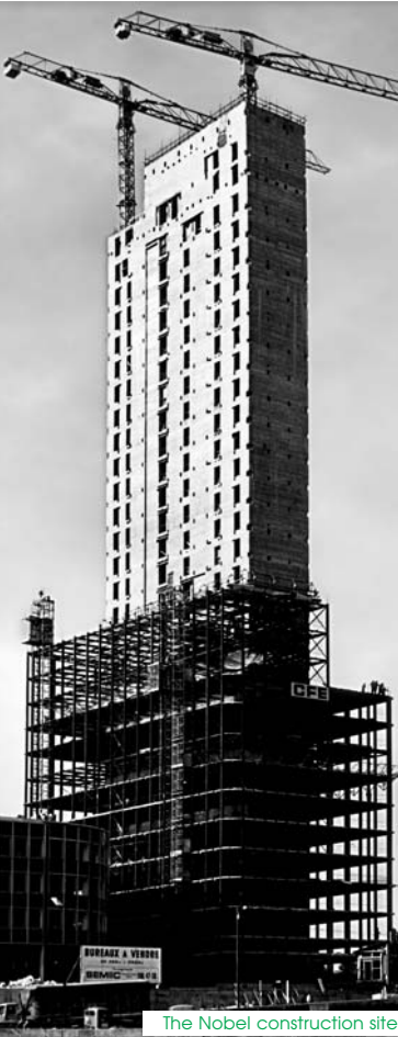
The Nobel construction site
